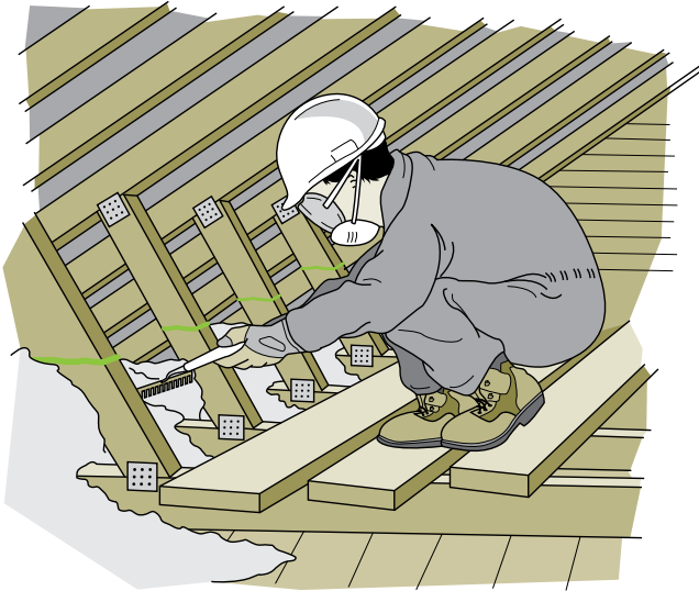
Figure 5-14 Installing loose-fill insulation
