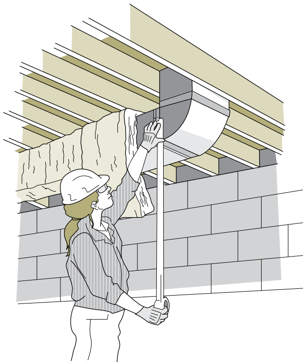
Figure 9-1 Taping an air duct
